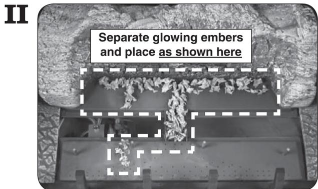
Separate a portion of the glowing embers into small pieces and evenly place them along the rear burner ports, ember screen, and front carry over ports as shown.
