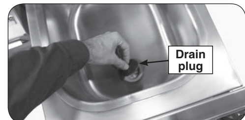
Fig. 7-4 Clean ice storage drain plug
