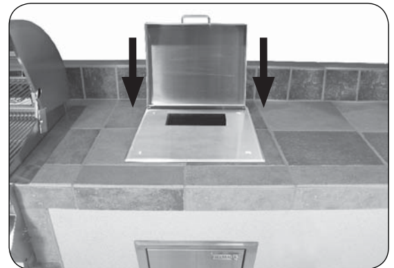
Fig. 3-2 Drop assembly into place
