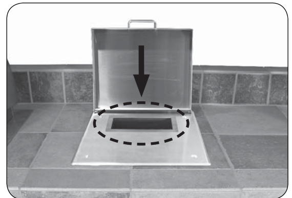
Fig. 3-3 Drop trash chute top into place
