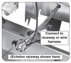
Fig. 5-3 Connect new electrode wires
