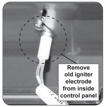
Fig. 7-1 Remove old igniter
