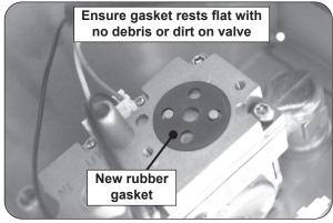
Fig. 5-1 Insert new rubber gasket
