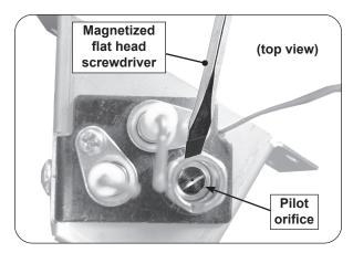
Fig. 3-1 Remove old and install new pilot orifice
