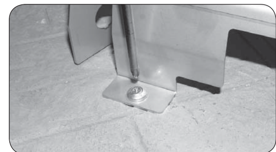
Fig. 9-4 Fastening hammer screws
