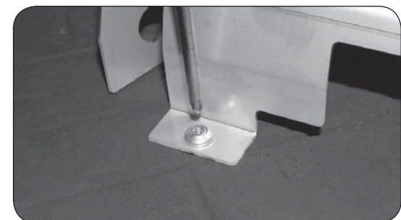
Fig. 9-4 Fastening hammer screws
