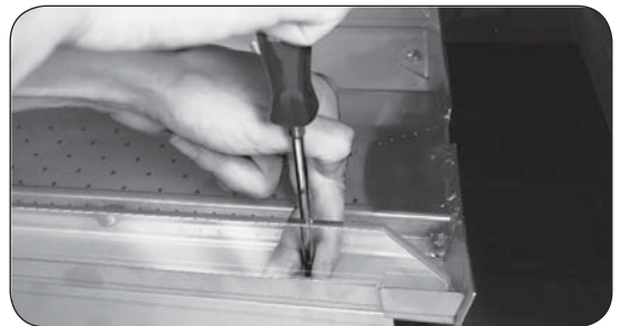
Fig. 7-3 Securing glass panel
