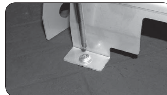
Fig. 6-4 Fastening hammer screws
