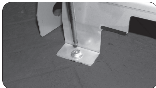
Fig. 10-2 Fastening hammer screws
