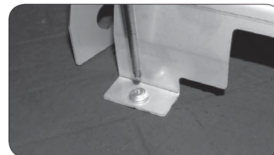
Fig. 6-4 Fastening hammer screws
