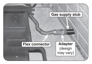
Fig. 8-2 Connect flex to gas supply
