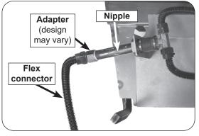
Fig. 8-1 Connect flex to burner
