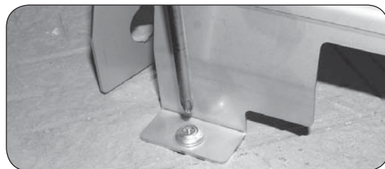
Fig. 15-3 Fasten hammer screws
