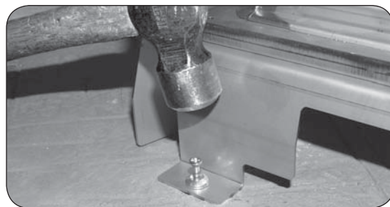
Fig. 15-2 Install hammer screws
