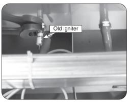
Fig. 2-1 Remove old igniter electrode
